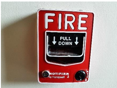
Fire Alarm Manual Station
