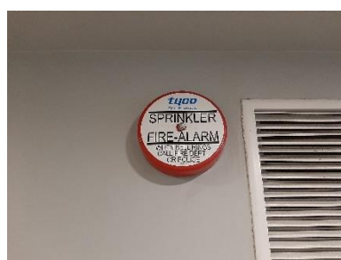
Sprinkle Fire Alarm
