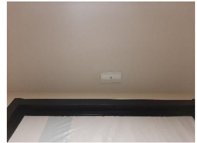
Fire Alarm Indicator Lamp
