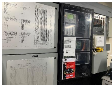
Graphic Annunciator Fire Alarm System
