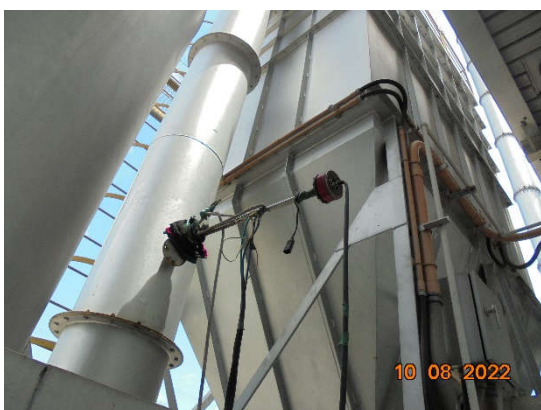
Bag Filter of Melting Furnace No.2 (S5)
