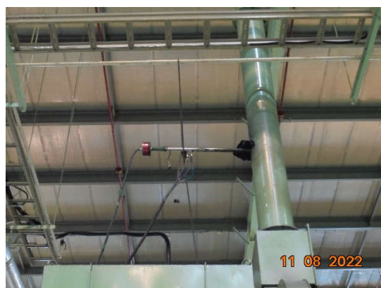
Bag Filter of Shot Blast Machine No.1 (S6)
