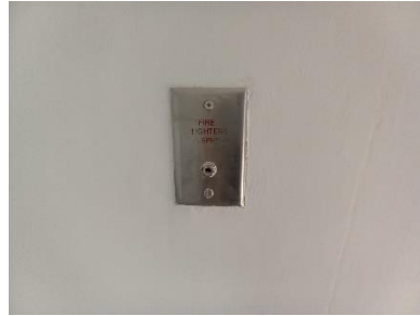
Fire Alarm Indicator Lamp
