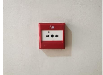
Fire Alarm Manual Station
