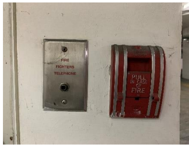
Fire Alarm Manual Station
