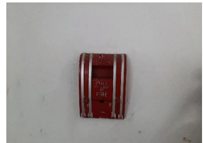
fire alarm manual station
