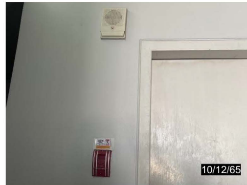
Fire Alarm Manual Station & Alarm Bell
