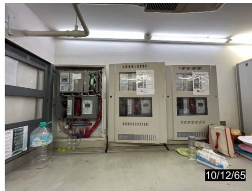
Fire Alarm Control Panel : FCP
