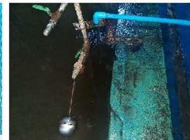
Level is high float not make up
