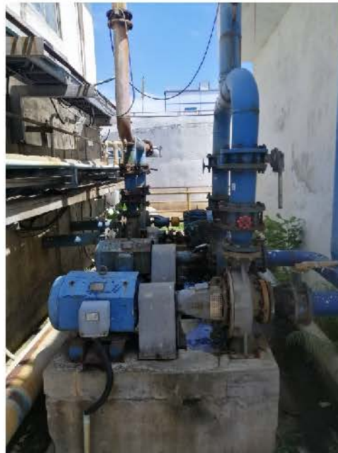
Service pump to re filter
