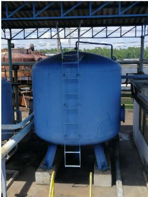
Sand filter tank
