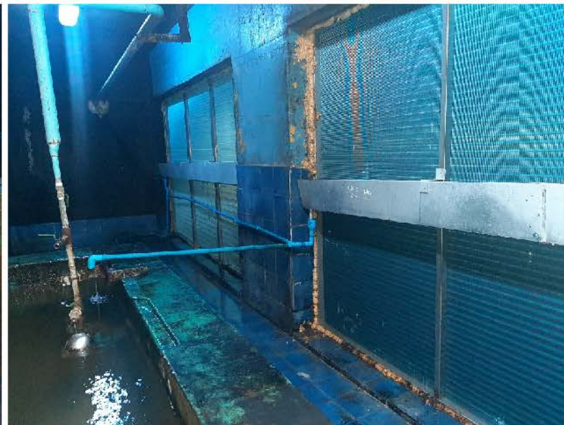
Tray , PVC pipe connect fill to pit
