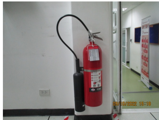
Portable Fire Extinguisher (CO 2 )
