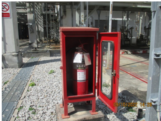
Portable Dry Chemical Extinguisher
