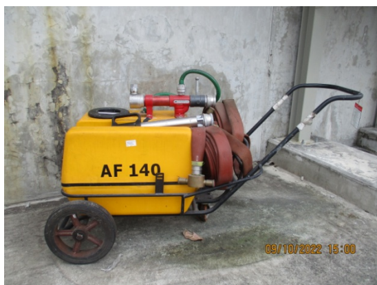
Wheel Foam Chemical Extinguisher
