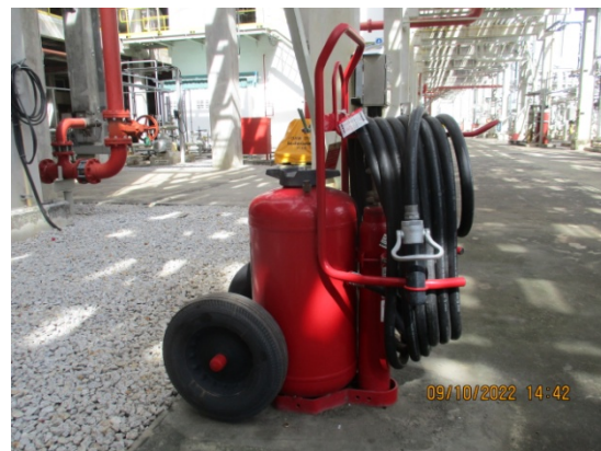
Wheel Dry Chemical Extinguisher
