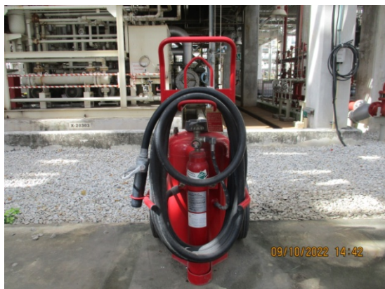
Wheel Dry Chemical Extinguisher
