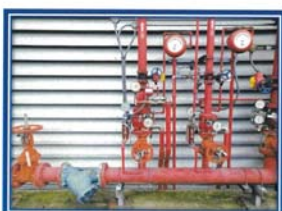
Picture shown : Return pre action system in normal condition.
