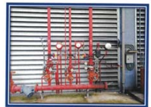
Picture shown : Inspection pre action system before function test.
