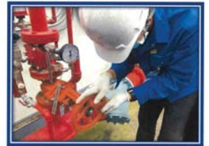
Picture shown : Reset deluge valve system after function test and return in normal condition.
