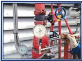
Picture shown : Function test low air pressure switch and control panel working properly.
