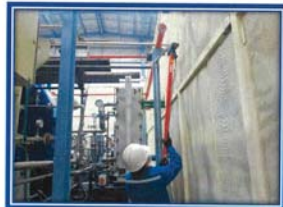
Picture shown : Function test heat detector of pre action system and control panel working properly.
