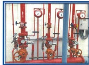
Picture shown : Return all deluge valve system at transformer area in normal condition.
