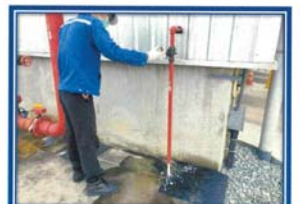
Picture shown : Function test automatic sprinkler system by drain test at Tripping Hall.
