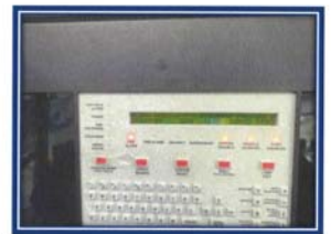
Picture shown : Function test alarm gong the pressure switch active at fire alarm control panel.
