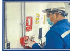
Picture shown : Function test manual call point at BOP Area and the device working properly.
