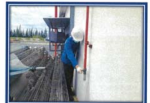
Picture shown : Function test automatic sprinkler system by drain test at Warehouse Building.
