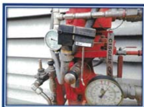
Picture shown : Function test crosszone and solenoid valve working properly.
