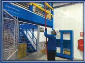
Picture shown :Function test smoke detector at Warehouse and the control panel working properly.
