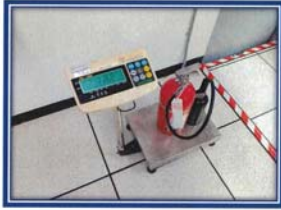
Picture shown : Inspection and weight check CO2 portable fire extinguisher.
