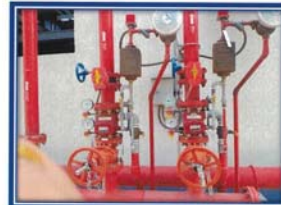
Picture shown : Function test automatic sprinkler system by drain test at Office Admin Building.
