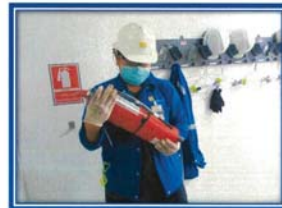
Picture shown : Inspection and check the dry checmical portable fire extinguisher.
