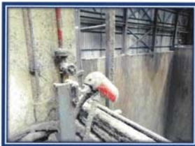
Picture shown : Inspection flame detector and remove out the device to testing at workshop.
