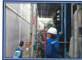
Picture shown : Function test heat detector of pre action system and heat detector working properly.
