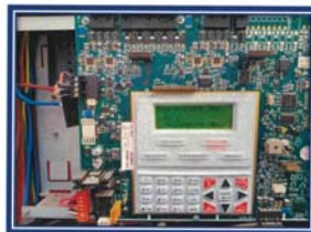
Picture shown : Function test low air pressure switch and control panel working properly.
