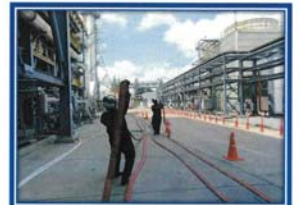
Picture shown : Picture shown : Hydrostatic test fire water hose.
