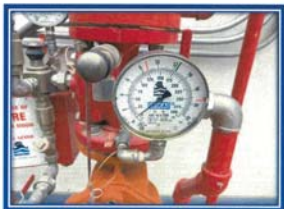
Picture shown : Function test manual release ball valve and the deluge valve working properly.
