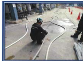
Picture shown : Maintain the pressure and inspect the fire water hose.
