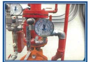
Picture shown : Return all deluge valve system at transformer area in normal condition.
