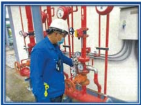
Picture shown : Function test manual release ball valve and the deluge valve working properly.
