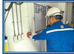
Picture shown : Function test manual call point at workshop area and control panel working properly.
