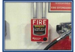
Picture shown : Function test manual call point at BOP Area and the device working properly.
