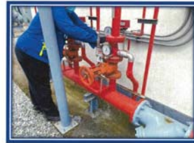
Picture shown : Reset deluge valve system after function test and return in normal condition.
