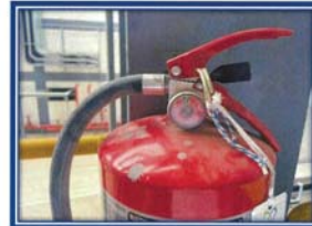
Picture shown : Inspection and check the dry checmical portable fire extinguisher.
