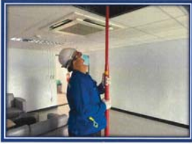
Picture shown :Function test smoke detector at BOP Area and the device working properly.
