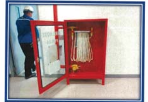
Picture shown : Inspection fire hose cabinet and fire hydrant.
