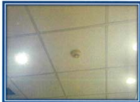
Picture shown :Function test heat detector and the device working properly.
