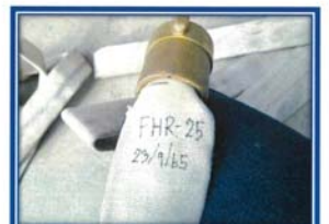
Picture shown : The fire hose No. FHR-25. leaked.
