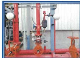
Picture shown : Function test automatic sprinkler system by drain test at Tripping Hall.
