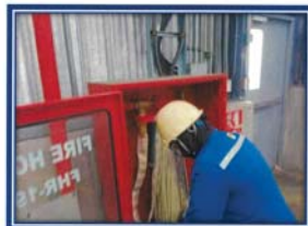
Picture shown : Inspection fire hose cabinet and fire hydrant.
