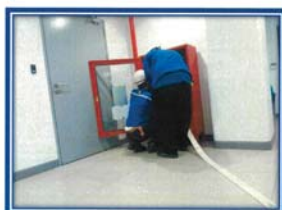
Picture shown : Inspection fire hose cabinet and fire hydrant.
