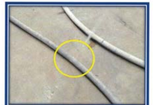
Picture shown : The fire hose No. FHR-18. leaked.
