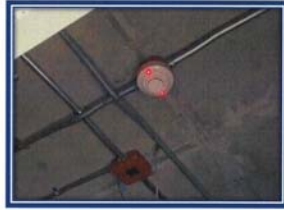
Picture shown :Function test smoke detector at BOP Area and the device working properly.
