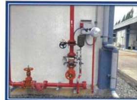
Picture shown : Function test automatic sprinkler system by drain test at Warehouse Building.
