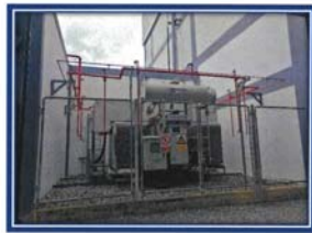
Picture shown : Inspection the deluge valve system at Transformer area 3 set.
