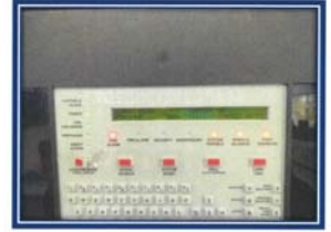
Picture shown :Function test heat detector at workshop area and the control panel working properly.
