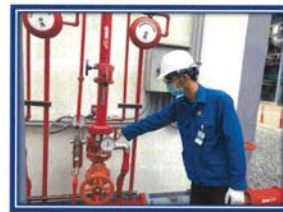
Picture shown : Function test alarm gong the pressure switch active at fire alarm control panel.
