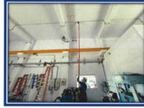
Picture shown :Function test heat detector at workshop area and the control panel working properly.
