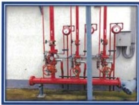
Picture shown : Inspection the deluge valve system at Transformer area 3 set.
