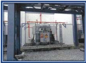
Picture shown : Inspection deluge valve system at Transformer area 3 set.
