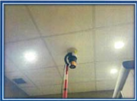
Picture shown :Function test heat detector and the device working properly.
