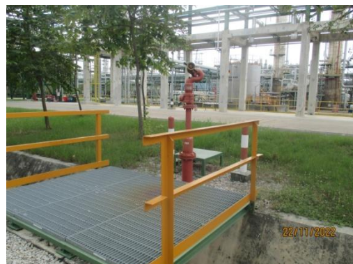
Water Hydrant with Monitor
