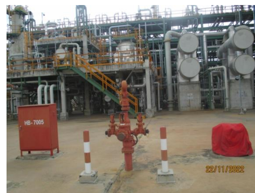
Water Monitor with Remote
