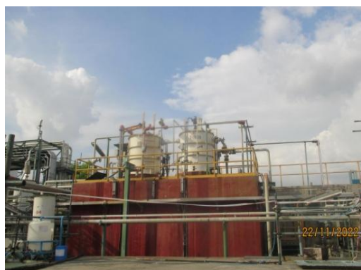
Neutralization Tank
