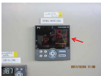
5. Stop make-up water pump at +170mm *Indication color will be red at \geq +170\text{mm} or \leq -170\text{mm}
