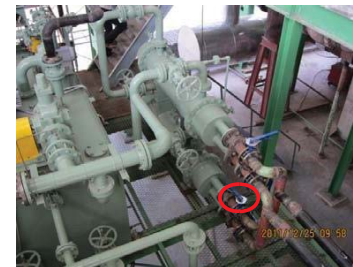
3. After 1 hour from vacuum break, close oil cooler cooling water outlet valve
