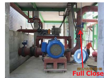
5. Stop cooling water pump after discharge valve full close
