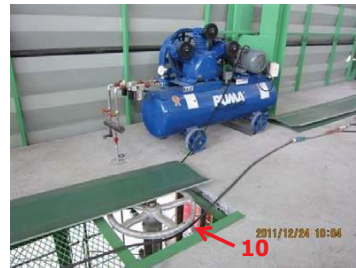
2. Close extraction steam isolation valve (10)
