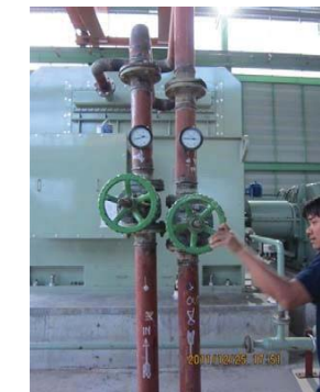
2. Close main steam isolation valve at distribution header
