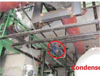
5. Check extraction drain trap isolation valve (to condenser) OPEN, and bypass valve CLOSE
