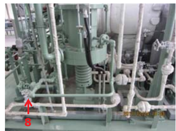
1. Open ESV drain valve (8)
