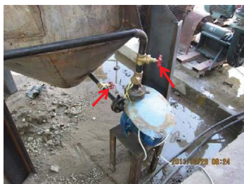
3. Check make-up water pump *Open valves
