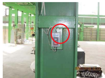
4. Start make-up water pump *Check hotwell level
