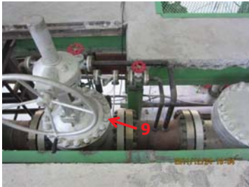
1. Close main steam isolation valve (9)
