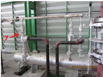
3. Close steam supply valve for 1st stage air ejector (7)
