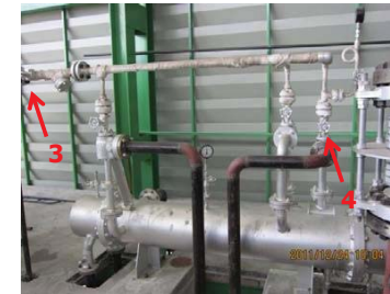
7. Close steam supply valve for gland ejector (4)
