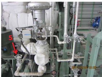
5. Wait until turbine exhaust steam pressure showing almost 0kg/cm2g
