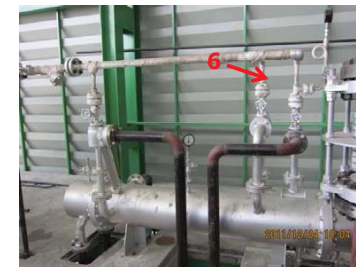
4. Close steam supply valve for 2nd stage air ejector (6)
