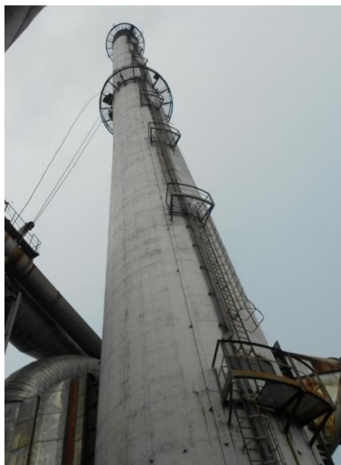
Combined Concrete Stack
