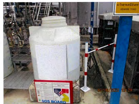
Sodium hydroxide tank (Boiler)
