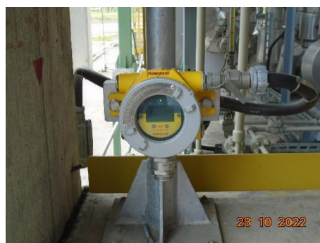
Gas Detector System
