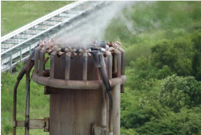
Figure 14: Flare Burner of elevated flare.
