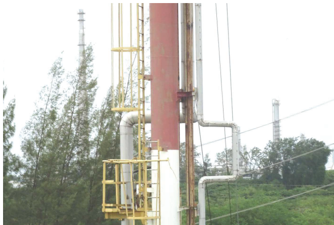
Figure 19: Omega pipe of flare.
