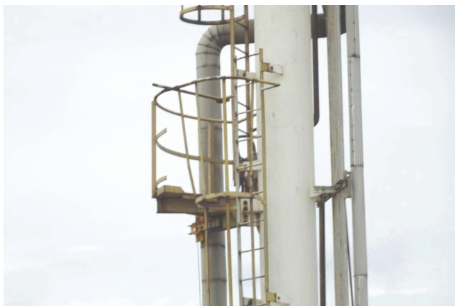
Figure 21: Omega pipe of elevated flare.
