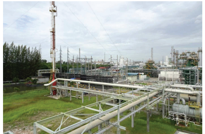
Figure 17: PP Process - Elevated Flare.
