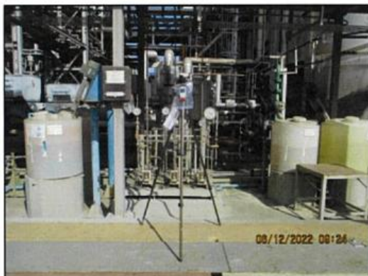
Chemical Feed pump (Phase 1)
