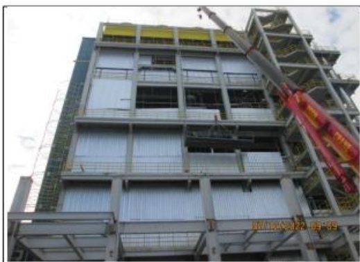
Installation Metalsheet Wall Protection
