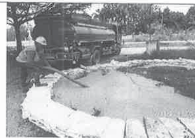
3) Suction truck Sucks Away Bentonite.
