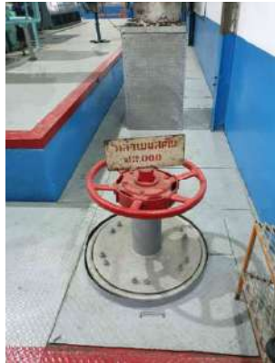
Bypass valve Turbine GEN.3
