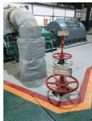
Bypass valve Turbine GEN.2
