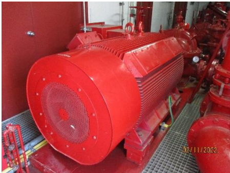
Electric Motor Driven Fire Water Pump
