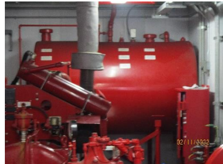
Diesel Engine Driven Fire Water Pump
