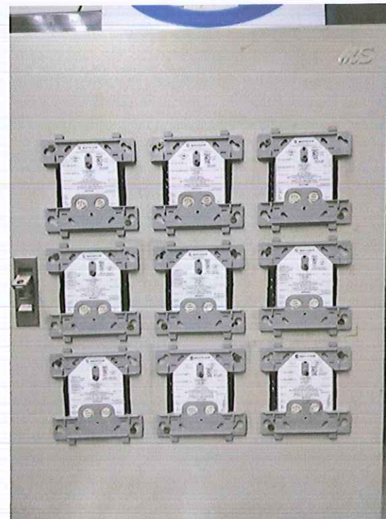
Fire Alarm Terminal Box (FATB) : Module
