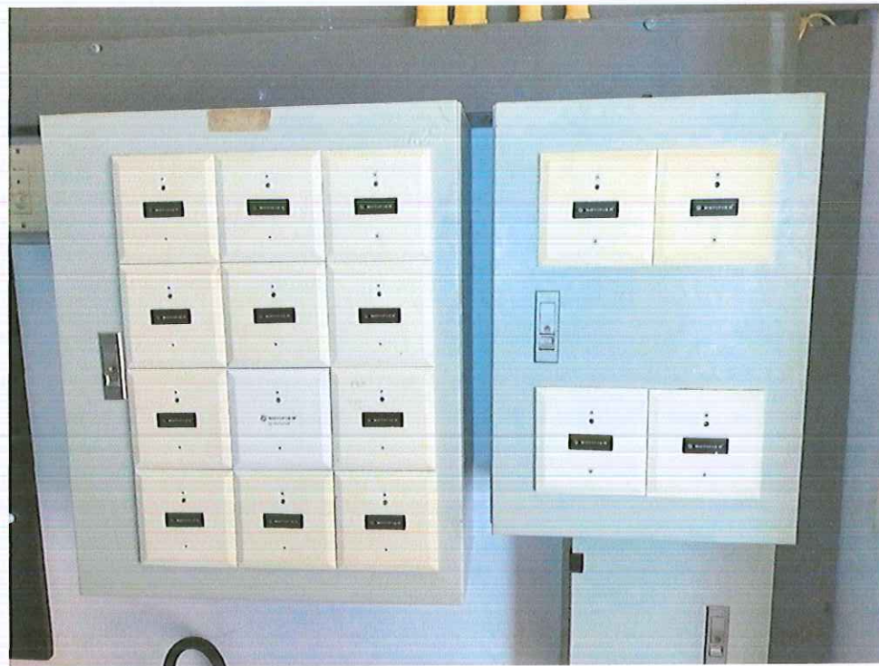
Fire Alarm Terminal Box (FATB) : Module
