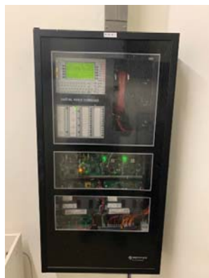
Fire alarm control panel
