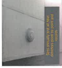
Smoke annunciator test all smoke and smoke light strobe by point and record
