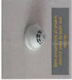
Smoke annunciator test all heat detector point by point and record
