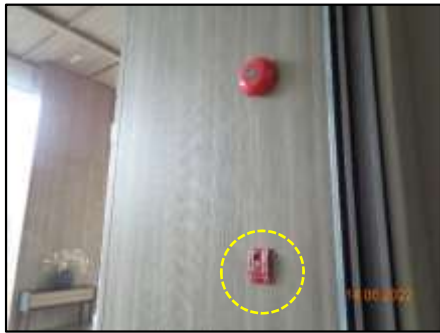
Fire Alarm Manual Station
