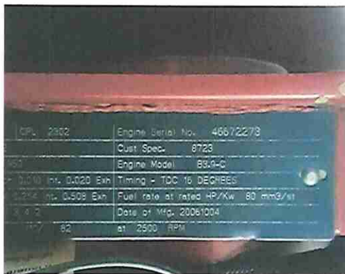
NAME PLATE ENGINE FIRE PUMP
