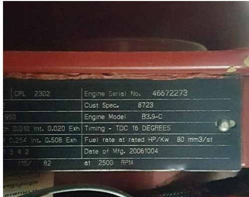
NAME PLATE ENGINE FIRE PUMP
