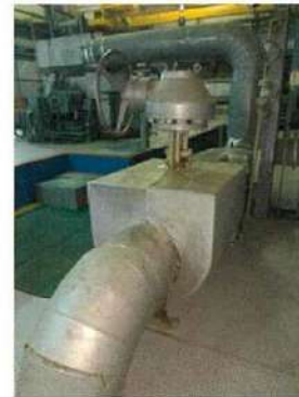
Pass valve Turbine GEN.4
