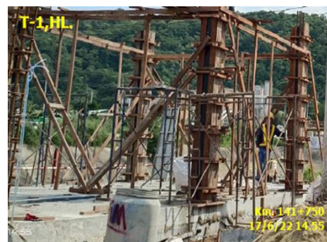
งาน Mechanical Building for Tunnel-Concrete Column
