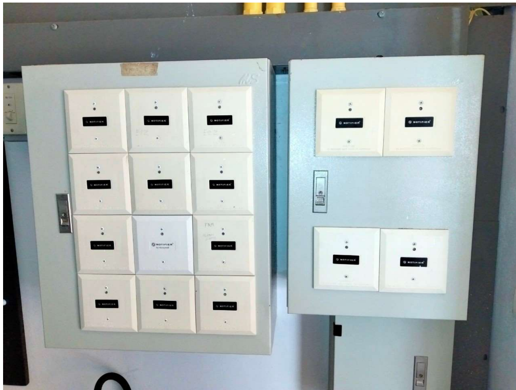
Fire Alarm Terminal Box (FATB) : Module
