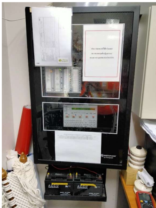
Fire Alarm Control Panel
