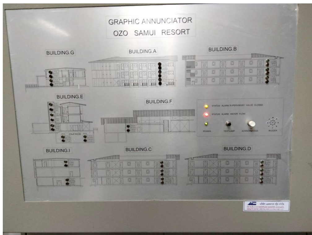
Graphic Annunciator for Fire Protection
