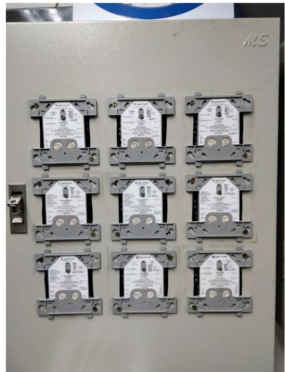
Fire Alarm Terminal Box (FATB) : Module
