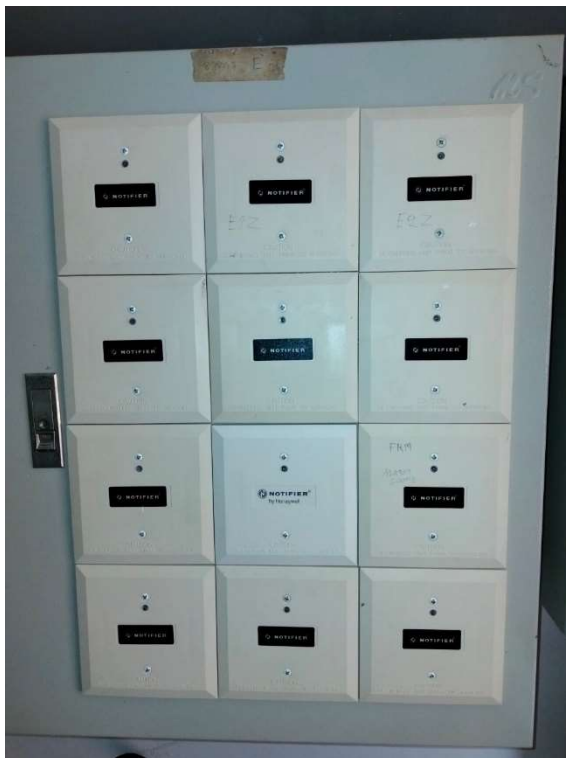
Fire Alarm Terminal Box (FATB) : Module
