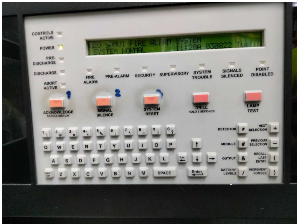
Fire Alarm Control Display
