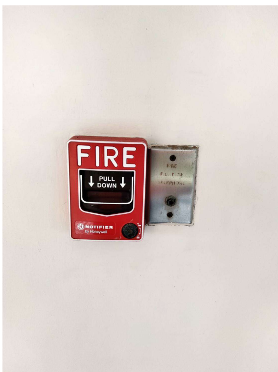
Manual Pull Station & Telephone Jack
