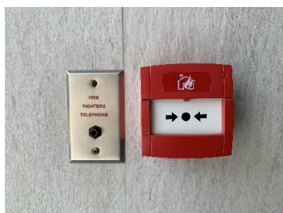
Fire Alarm Manual Station, Fireman Phone Jack
