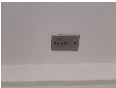
Fire Alarm Indicator Lamp
