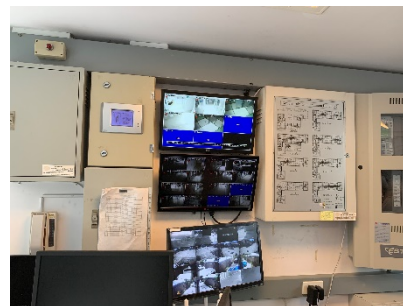
Graphic Annunciator Fire Alarm System
