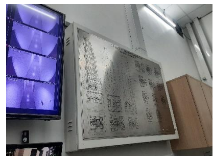
Graphic Annunciator Fire Alarm System
