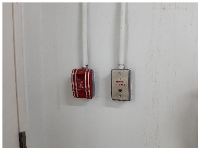
fire alarm manual station
