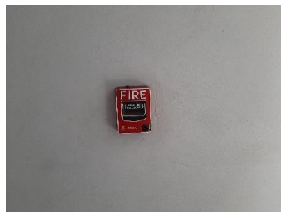
Fire Alarm Manual Station
