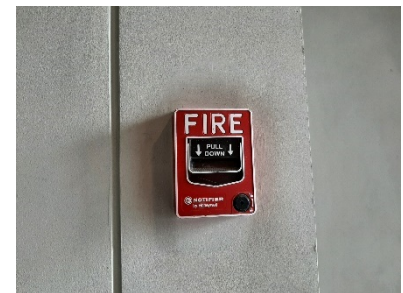
fire alarm manual station
