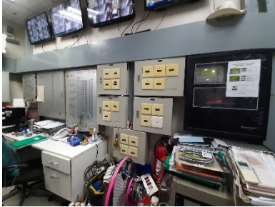
Graphic Annunciator Fire Alarm System
