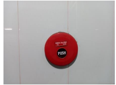
fire alarm manual station
