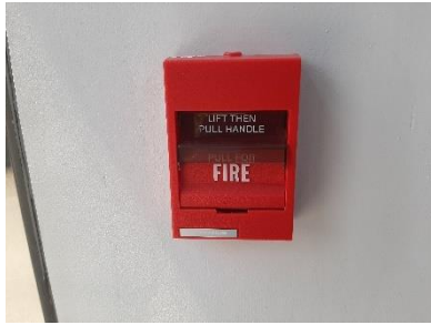
fire alarm manual station
