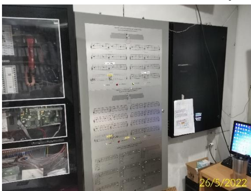
Fire Alarm Control Panel
