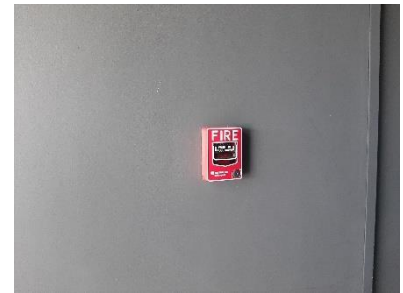
fire alarm manual station
