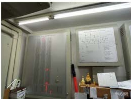
Fire Alarm Control Panel : FCP
