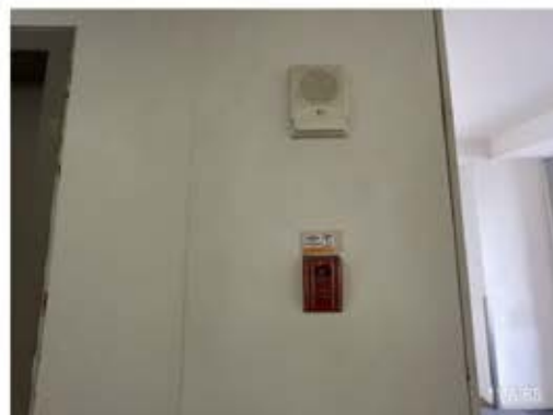
Fire Alarm Manual Station & Alarm Bell
