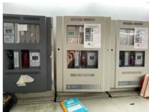
Fire Alarm Control Panel : FCP
