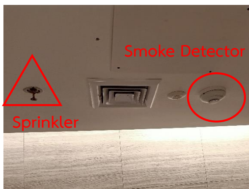
Smoke Detector & Sprinkler
