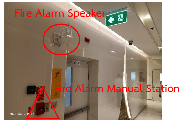
Fire Alarm Speaker & Fire Alarm Manual Station
