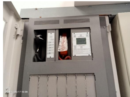
Fire Alarm Control Panel
