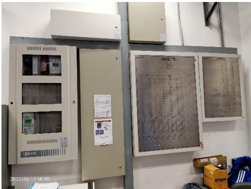
Fire Alarm Control Panel
