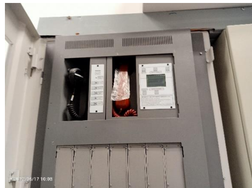
Fire Alarm Control Panel
