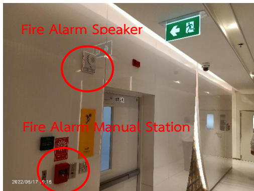
Fire Alarm Speaker & Fire Alarm Manual Station
