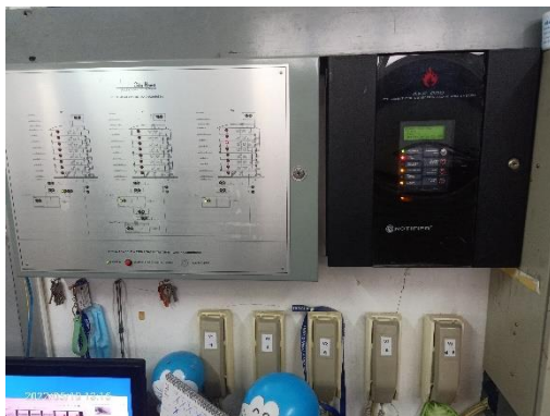
Fire Alarm Control Panel : FCP
