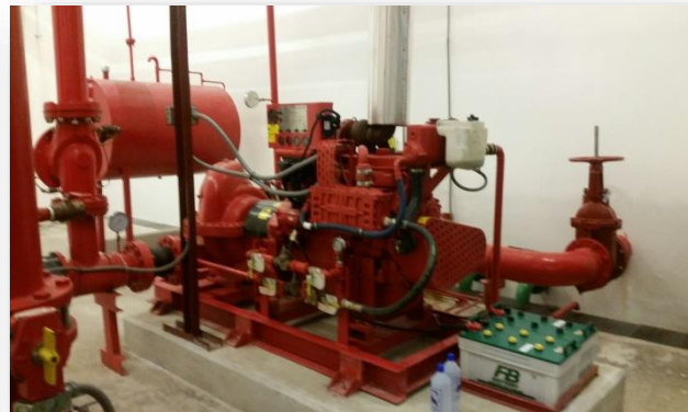
Diesel Fire Pump
