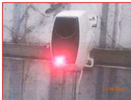
Smoke Beam Detector
