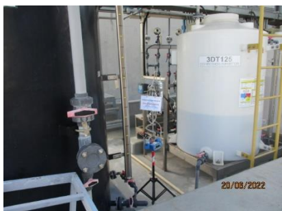
ABPR3_Chemical dosing (Cooling Tower 30)
