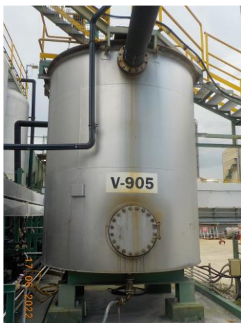
pH Control Tank (PC1)
