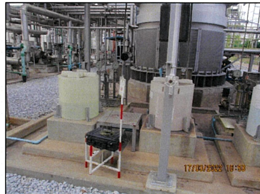
Chemical Feed Pump (Phase 4)
