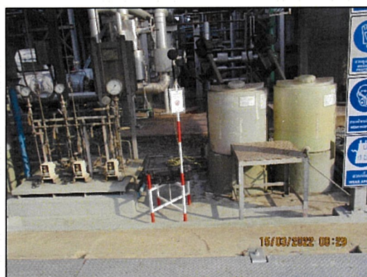
Chemical Feed pump (Phase 1)
