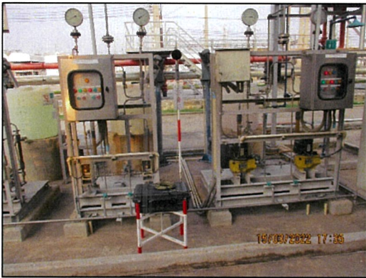
Chemical Feed Pump (Phase 2)
