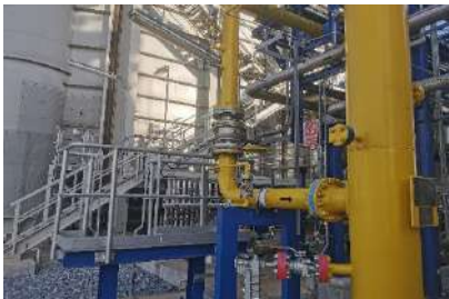
FG filter Block valve (isolate point2)
