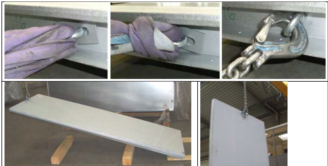
Fig.: 24 - Wall panel – Slinging and lifting with the crane
