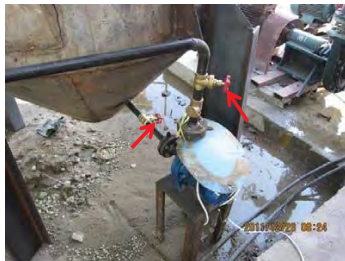
3. Check make-up water pump *Open valves
