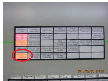
6. Level high alarm at +170mm
