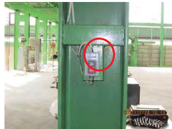
4. Start make-up water pump *Check hotwell level
