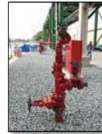
● Fire Hydrant with Monitor
