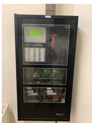
Fire alarm control panel
